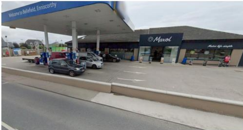
Photo taken from Google Street view August 2019
